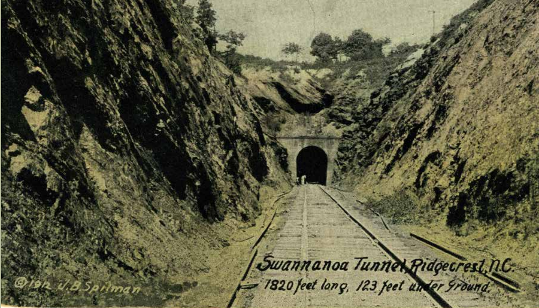
"Swannanoa Tunnel, Ridgecrest, N.C., 1820 feet long, 123 feet under ground" in Durwood Barbour Collection of North Carolina Postcards (P077), North Carolina Collection Photographic Archives, Wilson Library, UNC-Chapel Hill.
